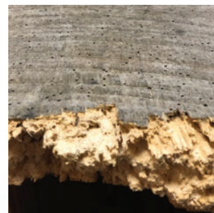
2x6 barn flooring destroyed by beetles
